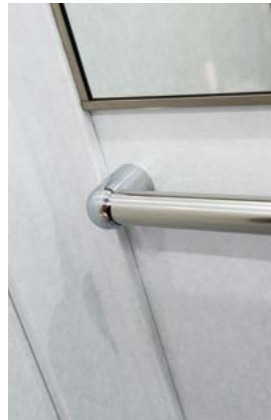
HANDRAIL: ROUNDED IN STAINLESS STEEL
